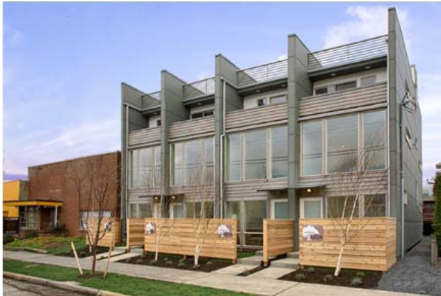
The Commission has financed the construction of more than 50 high-efficiency homes, including these built by Green Canopy Homes in Seattle.
